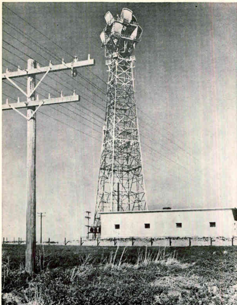
Typical relay station in Bell System's TH cross-country microwave network
