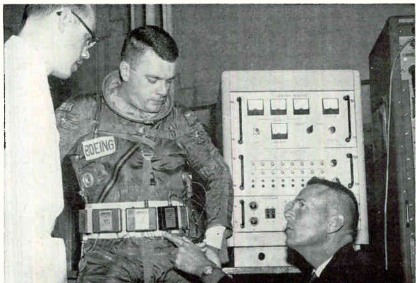
Miniature telemetering instruments, developed by Boeing for space medicine research, can be worn on belt, allowing subject to move freely. Arnoux Corp. will make the equipment
