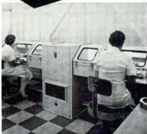
Acceleration tubes for Van-de-Graaff Particle Accelerators being assembled in the superclean atmosphere of Sterilshield Dust-free Workspaces at High Voltage Engineering Corp., South Bedford, Mass. The large unit in the center is a Model 1140 Sterilshield Air Cleaner, capable of servicing up to five Workspaces.
