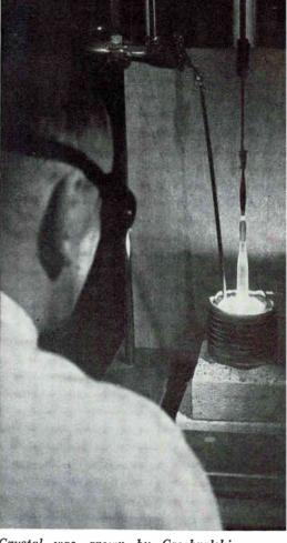
Crystal was grown by Czochralski technique. It is composed of calcium tungstate with trivalent neodymium
