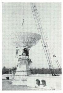
Reflector is lowered onto pedestal
