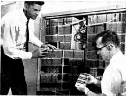
Holmdel Laboratory, N. J. We were developing an electronic switching system using new solid state devices. It will bring telephone customers a whole new range of services.
