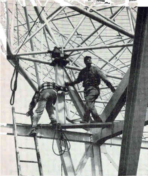
WORKMEN climb onto structure
