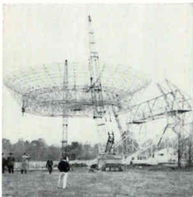
BIG DISH GOING UP. Huge cranes lift 63-ton radio telescope into position on towers at right. Reflecting surface of the 150-foot antenna is aluminum mesh
