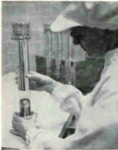
TUBE BODY is placed on elevator over target
