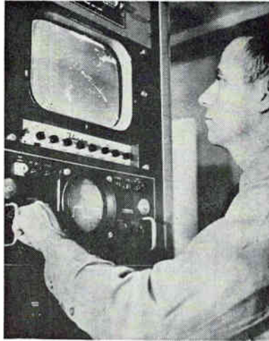
STORAGE TUBE is used to convert radar information into tv display in marine navigation aid
