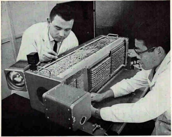
OPTICAL DECISION filter, developed by Astropower, using perceptron principles, recognizes three-dimensional geometric shapes. Wiring of associative networks is seen at top<sup>8</sup>
