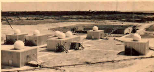
Azusa Mark II Tracking System at Cape Canaveral
