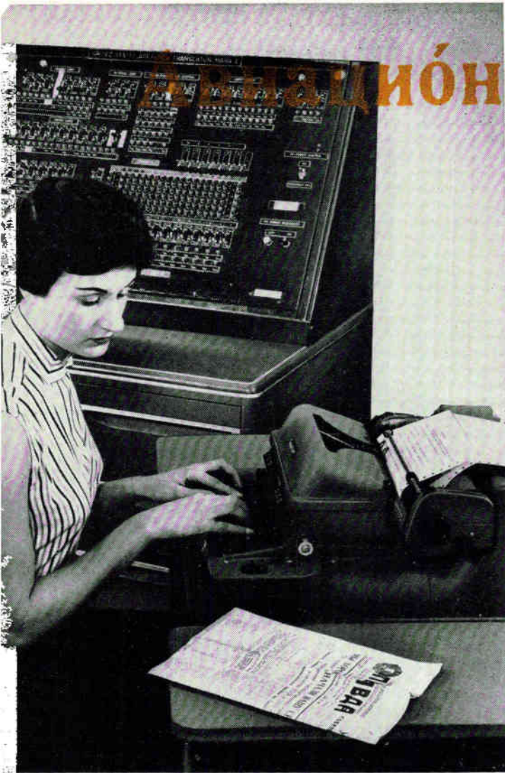
Typist copies an issue of Pravda on a special IBM electric typewriter which converts the Russian letters to punched holes in a paper tape. The tape is then read electronically and compared to Russian-English dictionary words stored on a ten-inch glass disk memory
