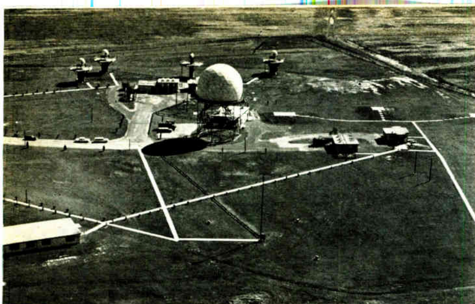
Improved Nike Hercules base in Maryland. Western Electric is prime contractor. GE built high-powered acquisition radar in large radome
