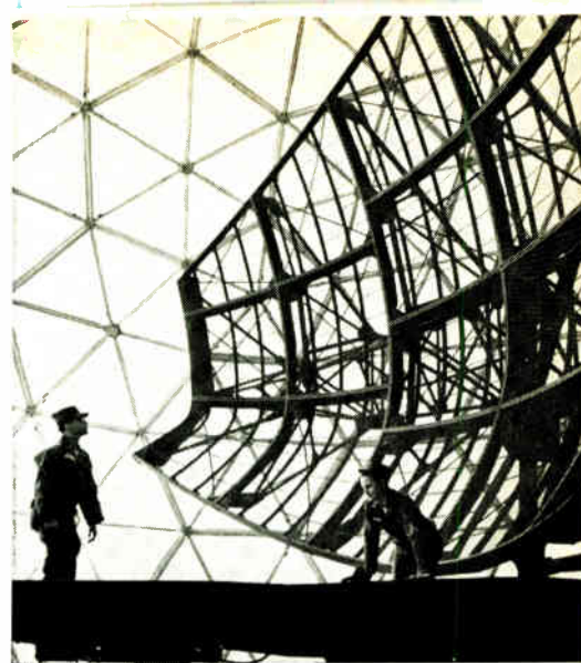
Inside the radome, Army missilemen check Hipar antenna
