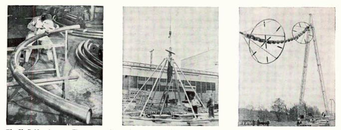
The U. S. Navy's two-million-watt radio station uses Republic Steel's stainless steel tubing to shield and grade the insulator string to prevent formation of corona and flashover. Top left photo shows welder joining a leg bracket to a section of grading ring. Center photo shows workmen attaching base plate to grading ring at Lapp Insulator's High Voltage Lab in LeRoy, N. Y. Rings and insulators are shown during final testing on dummy tower, right
