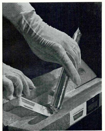
**Dow Corning single crystal** silicon is produced by vacuum zone refining hyper-pure polycrystalline rod. Result: The purest silicon produced! Typically, impurity content is only 0.15 part per billion of boron for crystals that are consistently above 1000-ohms centimeter resistivity. Boron content is even lower for crystals of 2000-ohms centimeter and above ... available on a selective basis.
