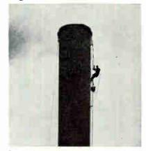
Corrosion check on chimney stack is made by field engineer in bosun's chair. He is using Magnaflux ultrasonic unit
