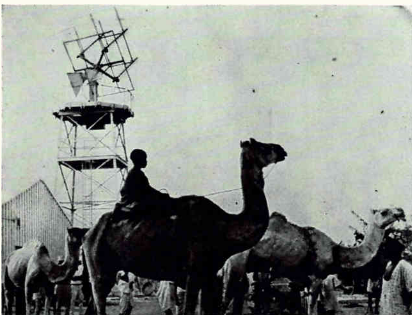
Agave antenna installed at Kano, Nigeria, by Cubic Corp. is part of Mercury network. This type of antenna picks up voice and telemetry signals as the capsule appears on the horizon and then tracks the spacecraft
