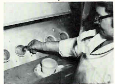
Wafers are polished in miniature barrel etchers
