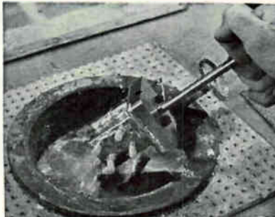
Master is dipped into pot of metal
