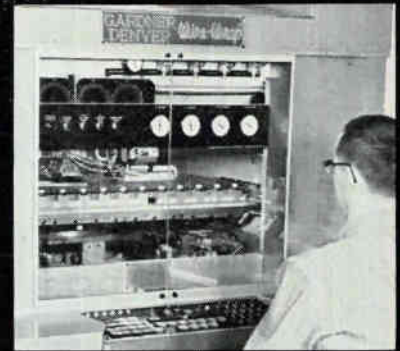
Gardner-Denver automatic "Wire-Wrap" machines expedite multiple operations.
