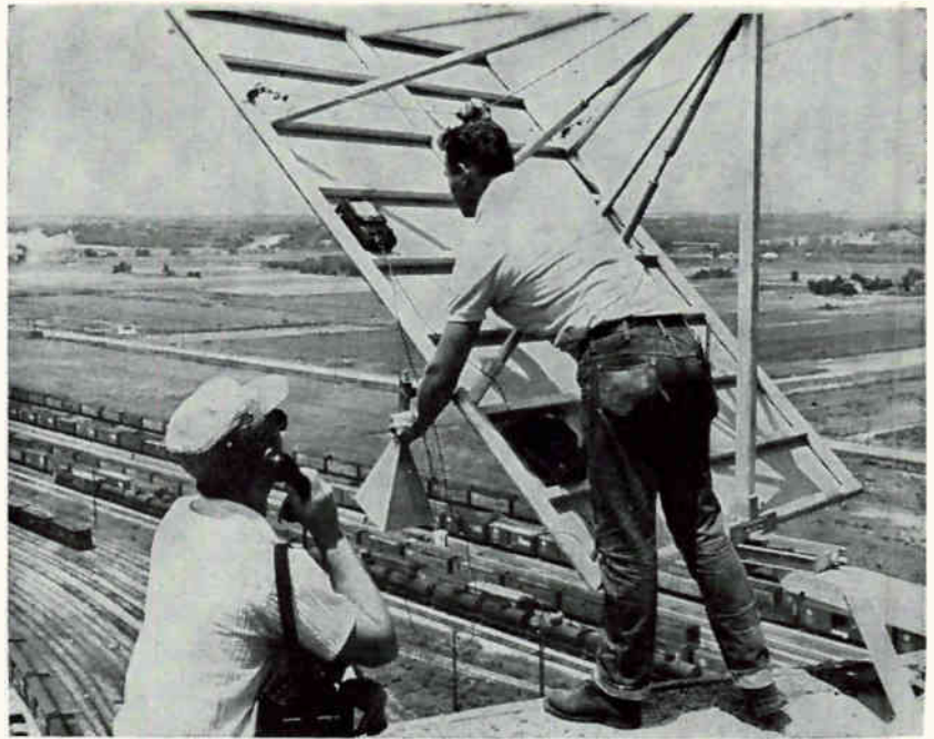
Santa Fe railway workers align a microwave antenna
