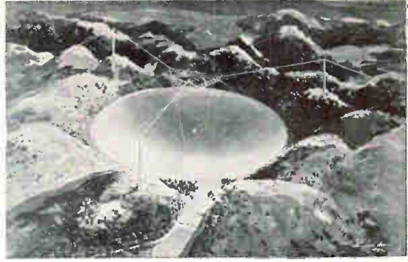
Natural bowl (left) in Puerto Rico will hold world's largest, most powerful radio telescope. Feed mechanism suspended above fixed dish will have capacity to rotate 360 degrees in azimuth and scan 20 degrees either side of vertical. Two of the towers now under construction will be 250 ft high and the third will be 365 ft
