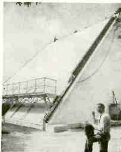
Project Defender's ESAR (electronically steerable array radar), Bendix, studies coasting missiles
