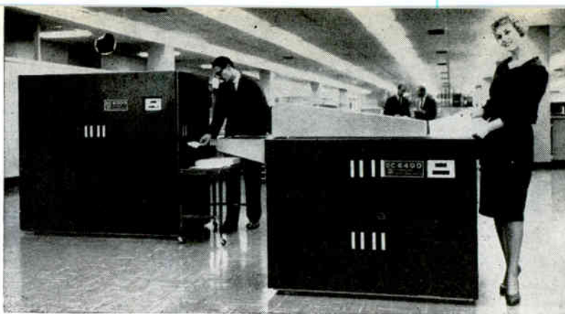
Type-written letter is transmitted digitally to xerographic printer at left using Stromberg-Carlson facsimile scanning and printing equipment
