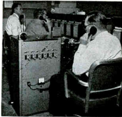
Chicago El line supervisor (foreground, left photo) flips control box switch and gets operating information from motorman aboard train
