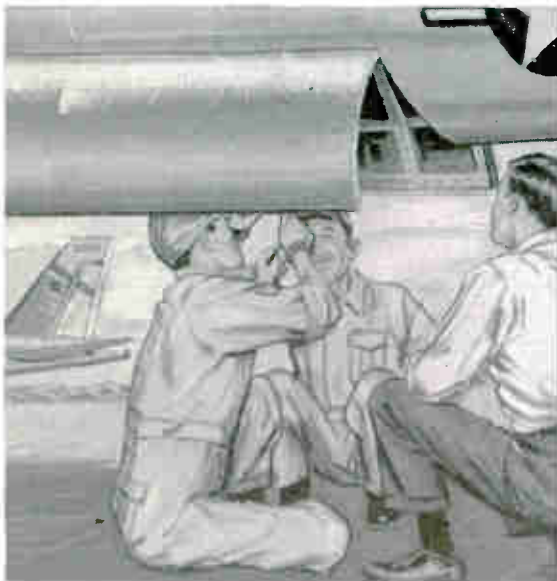
TEAMWORK IN MODIFICATION: Modernization of RF transmission systems completed in 30% less time through "BLUE STREAK" team assistance to base maintenance groups.
