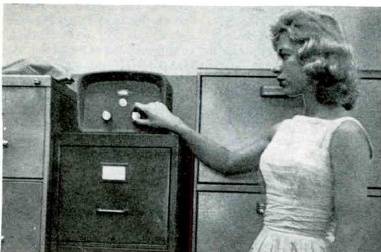
Typical installation shows alarm unit mounted on protected cabinets
