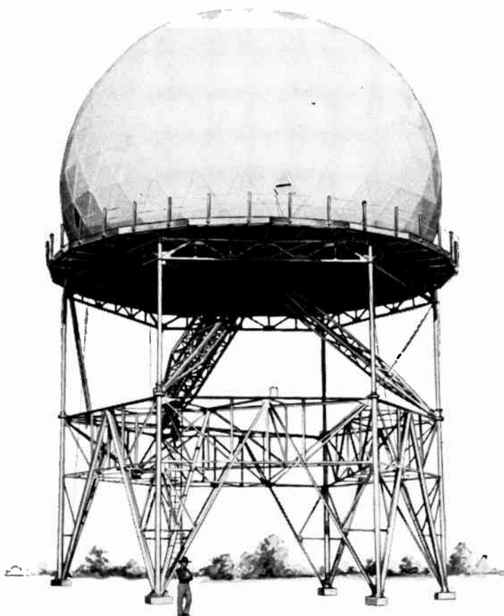
Fixed-Site Version of Improved Nike-Hercules Radar Tower incorporates the field army tower mounted on a 25' height-extension and fitted with a radome.
