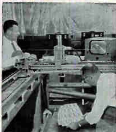
KinTel closed-circuit tv makes dimensional checks on aircraft components at Convair-San Diego
