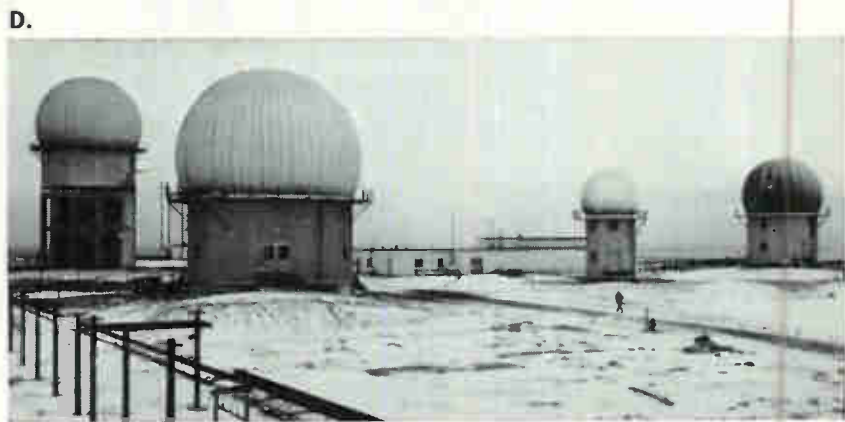
D. Surveillance radar towers on the DEW line. Designed for hurricane force winds and heavy ice and snow loads. These are some of more than 1,000 radar towers built by Dresser-Ideco for the nation's early warning systems.
