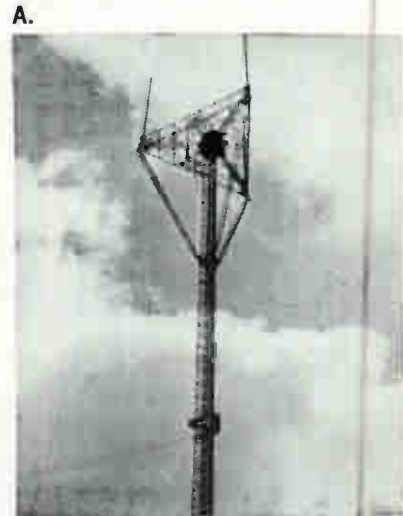
A. Multiple antenna tower. This big 729' tower in Baltimore supports three television antennas on a 105' wide platform at the top.
