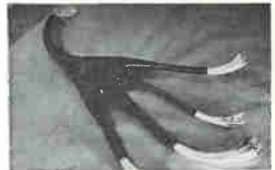
Finished cable junction
