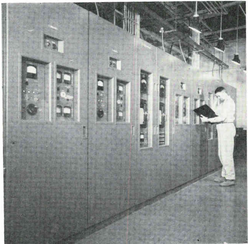
Power plant (2,800 volts) supplies the repeaters in the undersea cable. Instrumentation displays voltage and current fluctuations, amount of voltage each plant is supplying
