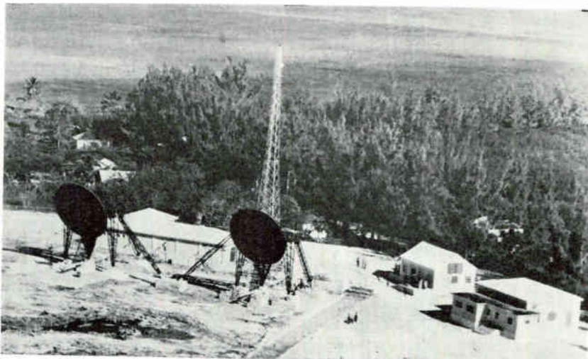
Nassau terminus of 186-mile over-the-horizon system, a joint project of AT&T and the Telecommunications Dept. of the Bahamas government. Linked with Florida City, Fla., the new system can carry 24 simultaneous telephone conversations. Total cost was $1½ million
