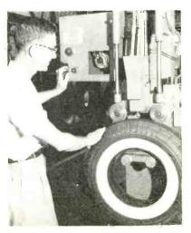
Variations in tire tread thickness are recorded at Goodyear electronics laboratory
