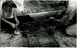
Fig. 2—Subbase contactors are installed prior to laying the pavement
