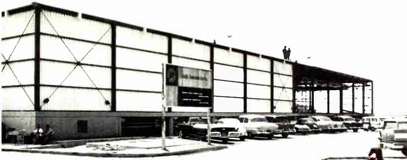
Close behind the bulldozers... a new home for PSI.
