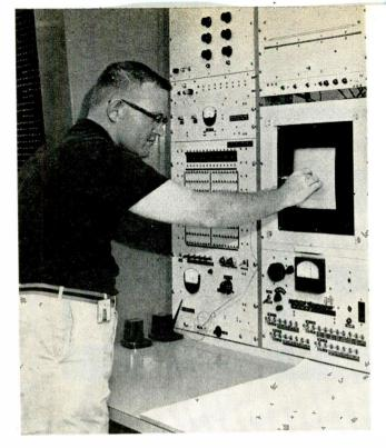
Operator reads crt display with pen-type sensor
