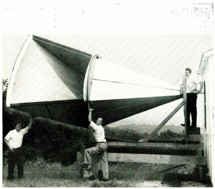
At Bell Laboratories, Holmdel, N. J., a korn reflector antenna is beamed skyward by scientists Edward Ohm, David Hogg and Robert DeGrasse. The maser amplifier, which employs a ruby cooled in liquid helium, is inside building at right. Over-all "noise" temperature of antenna, amplifier and sky is only 18°K at 5600 megacycles.
