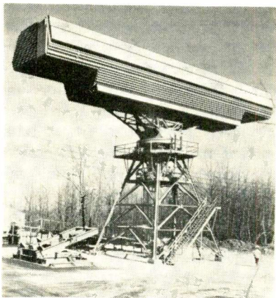
Rotating 50-ton radar antenna 104 ft long was developed for the Air Force by Raytheon. New antenna is designed for use with high power radars now undergoing final test
