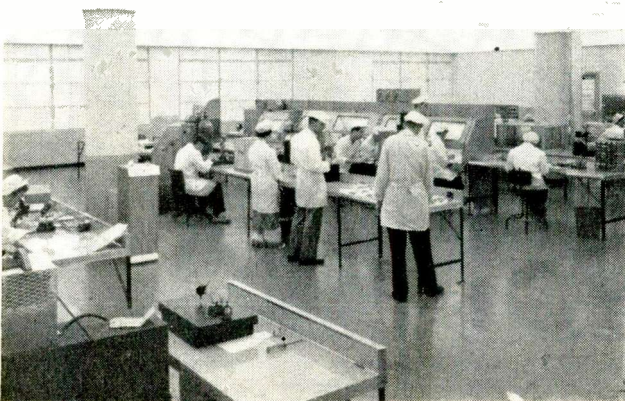
Portion of clean room built in former textile mill by Sanders Associates
