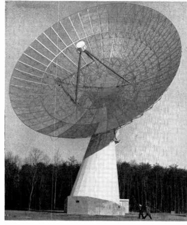
Naval Research Lab's 84-ft radio telescope at Riverside, Md., has maser at focal point<sup>.</sup>
