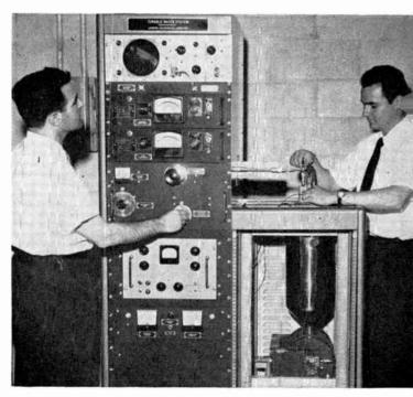
Engineers at Airborne Instruments Lab perform final tests on tunable L-band maser before delivery to Department of Defense
