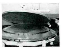
After curing, assembly is lifted off paraboloid face mold
