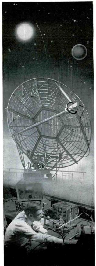
SIGNALS FROM PIONEER IV, 410,000 miles cut in space, were received at General Electric's tracking station at Schenectady, N.Y. using an 18' parabolic antenna having a 32 db gain and a parametric amplifier employing a Microwave Associates Varactor with a noise figure of 1 db.
