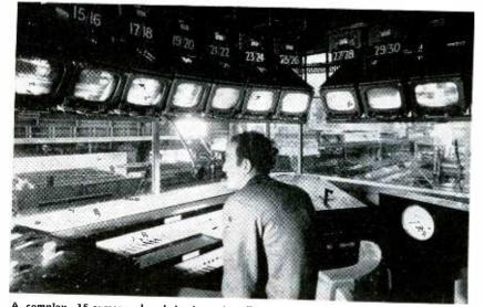
A complex, 15-camera closed-circuit tv installation helps speed output at Steel Company of Wales, Port Talbot, Wales. Marconi's Wireless Telegraph Co. Ltd. placed cameras in a line on one of rolling mill's outside walls. Operator gets composite view of 700 ft of track, far end of which is 1,000 ft away
