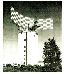
New experimental high-power search radar, designed by MIT's Lincoln Laboratory, is operating in North Andover, Mass. Radar reportedly has frequency of 400 mc with peak power of 5 megawatts. Reflector: 120 ft wide, 30 ft high
