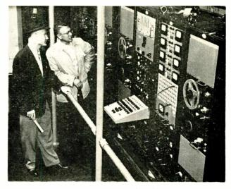
Telemetry recorders on downrange picket ships
