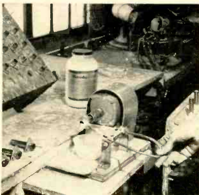
Shaped parts rotate between brushes loaded with flux
