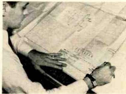
First step is preparing vellum pasteup of repetitious detail cut from an expanded drawing
