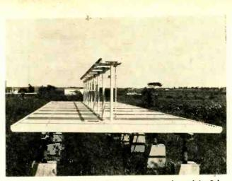
Closeup view of one of the Minitrack antennas located in Cuba. In the background is the ground-station trailer
