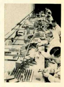
PROTOTYPE QUANTITIES of printed wiring boards are assembled at Avco's Advanced Research and Development Division, Lawrence, Mass., on small assembly lines like the one shown. In addition to purchased fixtures and feed trays, the assemblers are using 2 fixtures made in the division's shops.
