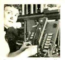
Slots keep wires sorted out after soldering to connectors
