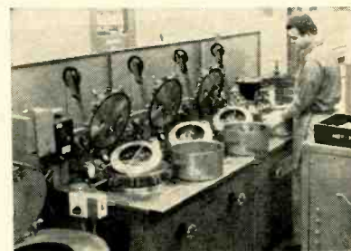
Each basket holds 4,000 disks in vacuum impregnator
