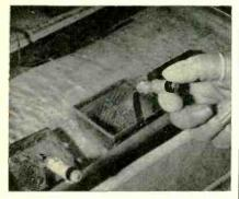
Transistor assemblies are placed in wire baskets for easy handling in cascade
