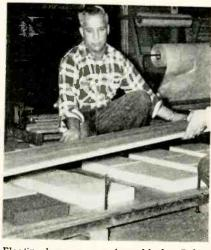
Floating base goes on foam blocks. Bolts in base are capped with springs
