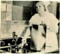
DRIED BLOOD, bits of tissue and other soils on surgical instruments are removed by cavitation caused by ultrasonic sound waves (upper photo) generated in a new medical washing machine (lower photo) manufactured by Acoustica Associates, Inc., of Mineola, N. Y.
