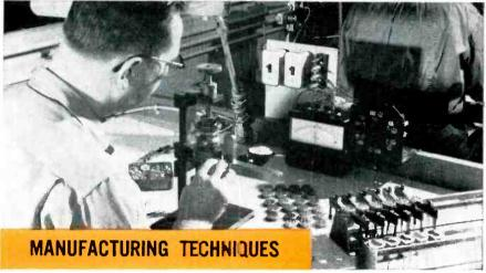
To obtain reliable performance in every relay, UNION has developed excellent techniques for precision manufacture on a high-volume basis. Workers are provided with ingenious tools, jigs and fixtures for consistent accuracy. Special processes such as high-temperature baking and hermetic seal by welding of steel cases assure top relay performance.
