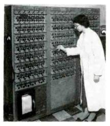
Sample transistors are operated in these racks from 500 to 2,000 hours at Delco Radio division of General Motors
