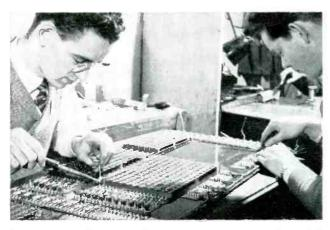
Several connections on redundancy table must be changed for each draw to include bond numbers issued since previous draw
