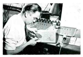
Printed wiring boards are equipped by hand. Terminals at end permit rewiring to provide other counter and storage facilities
