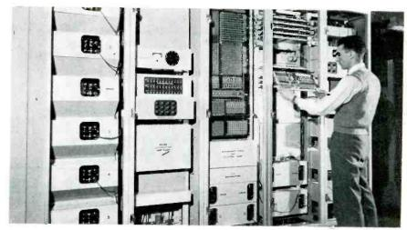
Printed wire panel of master control is tested at left. Overall view of right shows hand-wired redundancy able in center
