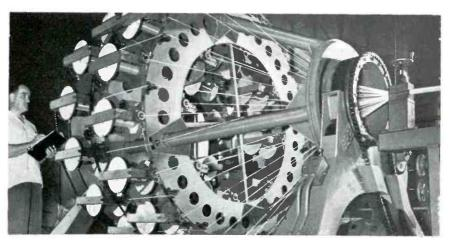
Producing complete umbilical-cord cable for guided missile on model D-100 Douglas planetary cabler. The two rings of wire reels rotate in opposite directions to give a contrahelical lay, and each reel tumbles about its own transverse axis while unreeling to remove twist from conductors
