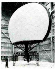
**COLLAPSIBLE** magnesium base aids mobility of this new portable paraballoon radar antenna with an inflatable reflector, developed by Westinghouse for the Air Force as . . .
