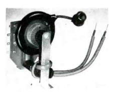
Complete transformer using coil having new protective butyrate tire
