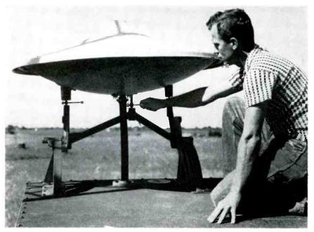
Electronic equipment at various repeaters is housed in transportable shelters on which are mounted microwave antennas such as that being adjusted here
