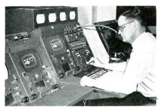
Operator punches up call-letter slide on switching-mixing unit
