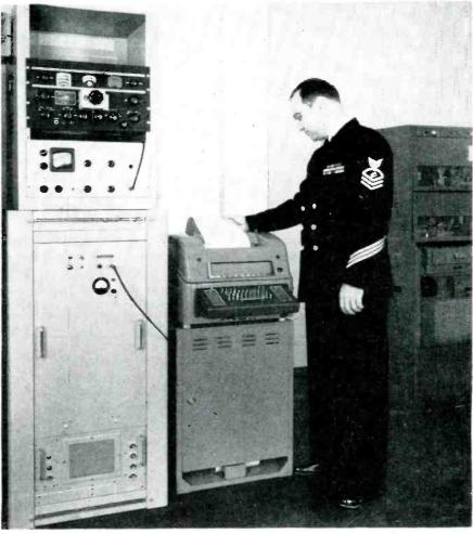
Trak model CMP-15 Morse-to-teleprinter code converter (lower left) installed for evaluation at U. S. Navy Radio Station, Cheltenham, Md., with station WWL being copied by interconnected Teletype machine at 100 words per minute. Radio receiver and static rejector are in rack above converter.—Official photograph, U. S. Navy
