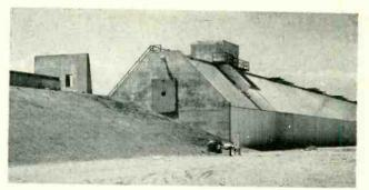
Ordnancemen load one of guns on mound outside laboratory. Projectile is fired through rectangular hole into Aeroballistics Laboratory, shown at right, in which range stations are located
