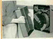
Wall-mounted Type W50M. Four 1½" conduit knockouts provided for convenience in wiring. Four bolts through comers of base and case attach W50's to wall or panel – 2 screws in top hold cover firmly in pace — captive radiator permits shaft to be extended either way for panel or wall mounting without upsetting radiator and brush setings. Note accessibility of terminal board for easy wiring.
