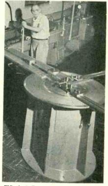
FIG. 6—Pulling mandrel out of tubing after 90-deg bend with ½ inch-radius
