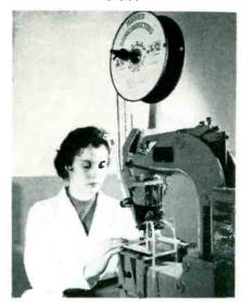
Ammunition belt feeds 3,000 semiconductors into machine that staples them into electronic circuits at Hughes Aircraft. A special machine was developed to fabricate the belts
