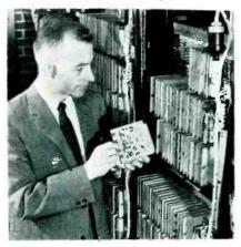
Plug-in type camputer uses printed circuits, 1,500 transistors and 11,000 diodes as part of radar track-while-scan system that automatically tracks up to 72 targets in three dimensions. Developed by Westinghouuse, the system presents three-dimensional information from a single-radar source
