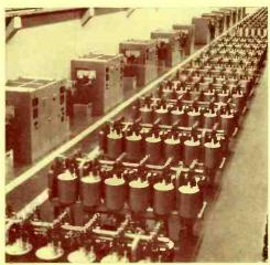
LEFT: a continuous air-tight weld of ignitron covers to tanks is formed by rotating the big tubes in motorized jigs. RIGHT: showing a large rectifier installation of G-E pumpless ignitrons. Note the clean layout, free from vacuum pumping equipment, headers, gages, and connections. Eliminating these components saves substantially in equipment, power, and maintenance costs.
