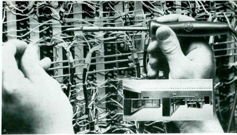
NEARLY 500 G-E MIDGET SOLDERING IRONS are helping to speed assembly of IBM's giant 704 and 705 "electronic brains" by providing fast, efficient heat to thousands of intricate joints. Each complex data processing machine demands perfectly soldered joints to assure dependable operation. IBM found that the G-E Midget irons provide excellent heat recovery, even with
