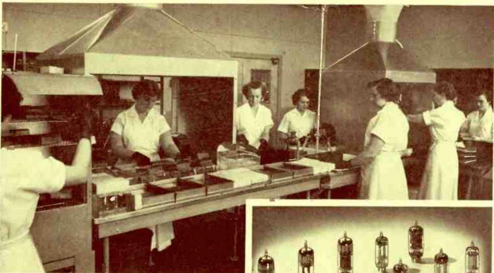
Conditioned air, pressurized to keep out dust and dirt; lint-free Dacron garments; gloved hands . . . these accent the surgically clean conditions that apply when cleaning grids of the ten G-E computer tubes shown at lower right.
