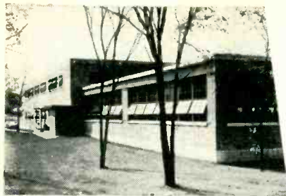
▲ Plant of Westchester manufacturing subsidiary, Pleasantville Instrument Corporation; additions are under construction.
