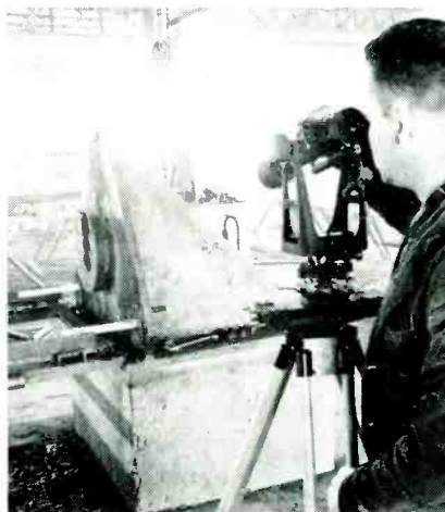
Checking base plate No. 1 with first jig transit
