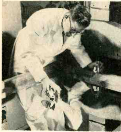
SUBMICROSCOPIC iron particles are collected from a pool of liquid metal with a conventional magnet (left). These are later pressed to form a superpower magnet that can be drilled and tapped as . . .
