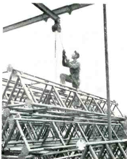
Examples of tower sections welded with aid of precisely aligned fixture
