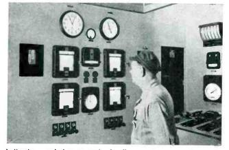
Indicating panel of power station has linear and circular self-balancing recorders to record steam-gas and air, feedwater and other temperatures on continuous basis
