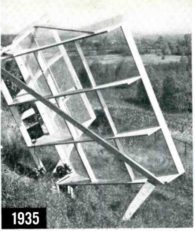
EARLY RESEARCH AND DEVELOPMENT EXPERIENCE with electronic location equipment at G.E. began in 1935 when this first system, with an output of  $1\frac{1}{2}$  watts, located planes up to five miles away.
