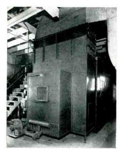
A Type CH Lectrodryer like this does the DRYing.
