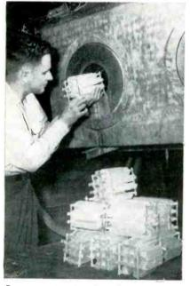
Removing batch of half-pound grown quartz crystals from Clevite autoclave. All crystals ore essentially identical in shape, weight and orientation
