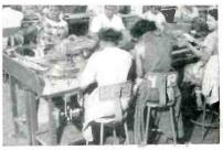
Folded assembly line for i-f subassemblies, showing one of the six pass-along bends in the two-track line
