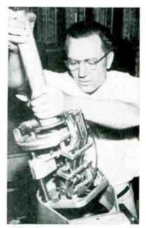
Removing insertion head
