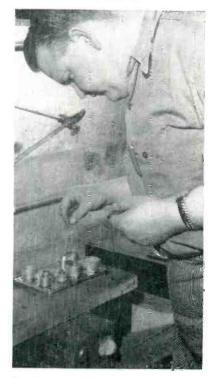
Touching up soldering on hot plate
