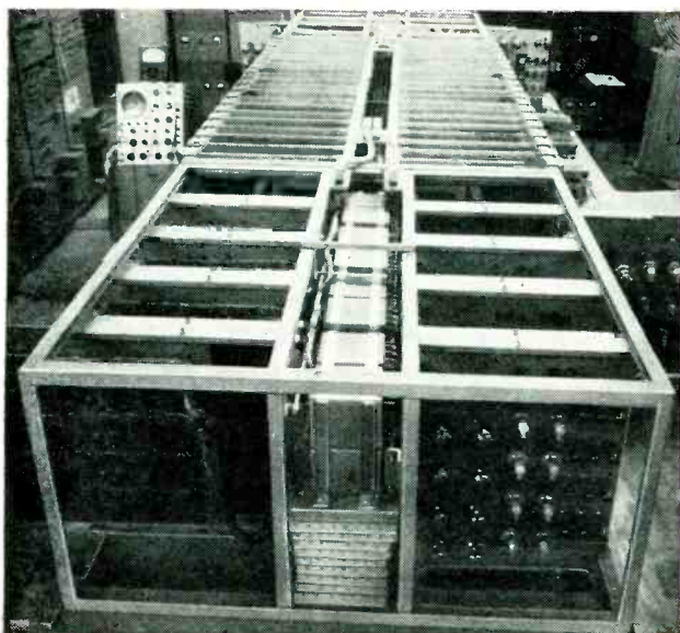
Ferrite-core memory is designed for JOHNNIAC computer
