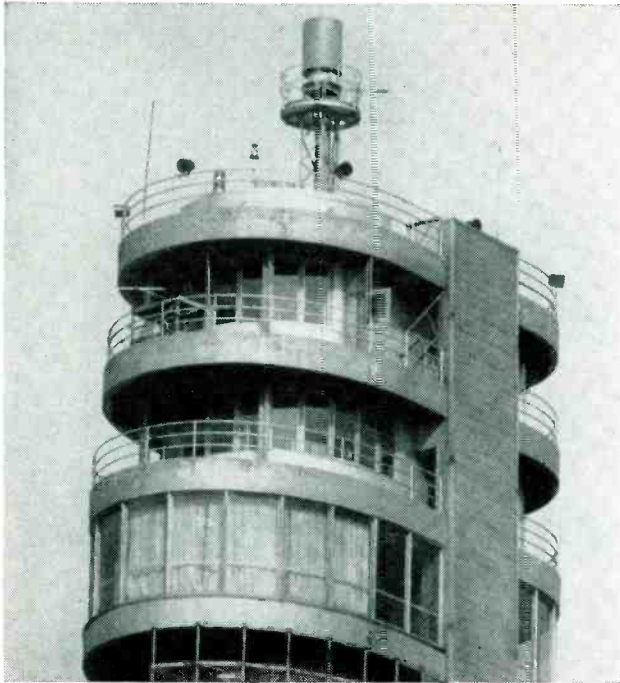
Experimental TACAN antenna atop 300-ft tower
