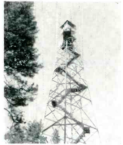
Cabin on Mt. Danaher lookout tower is 100 feet above ground
