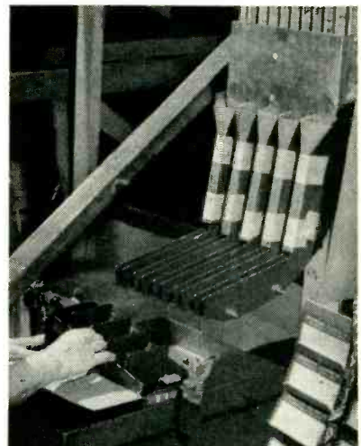
Placing separator frame in empty carton that rests on top of shaker mechanism
