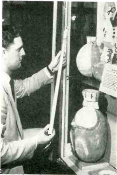
Ribbon-type transducer placed at side of display case sets off alarm if objects are moved
