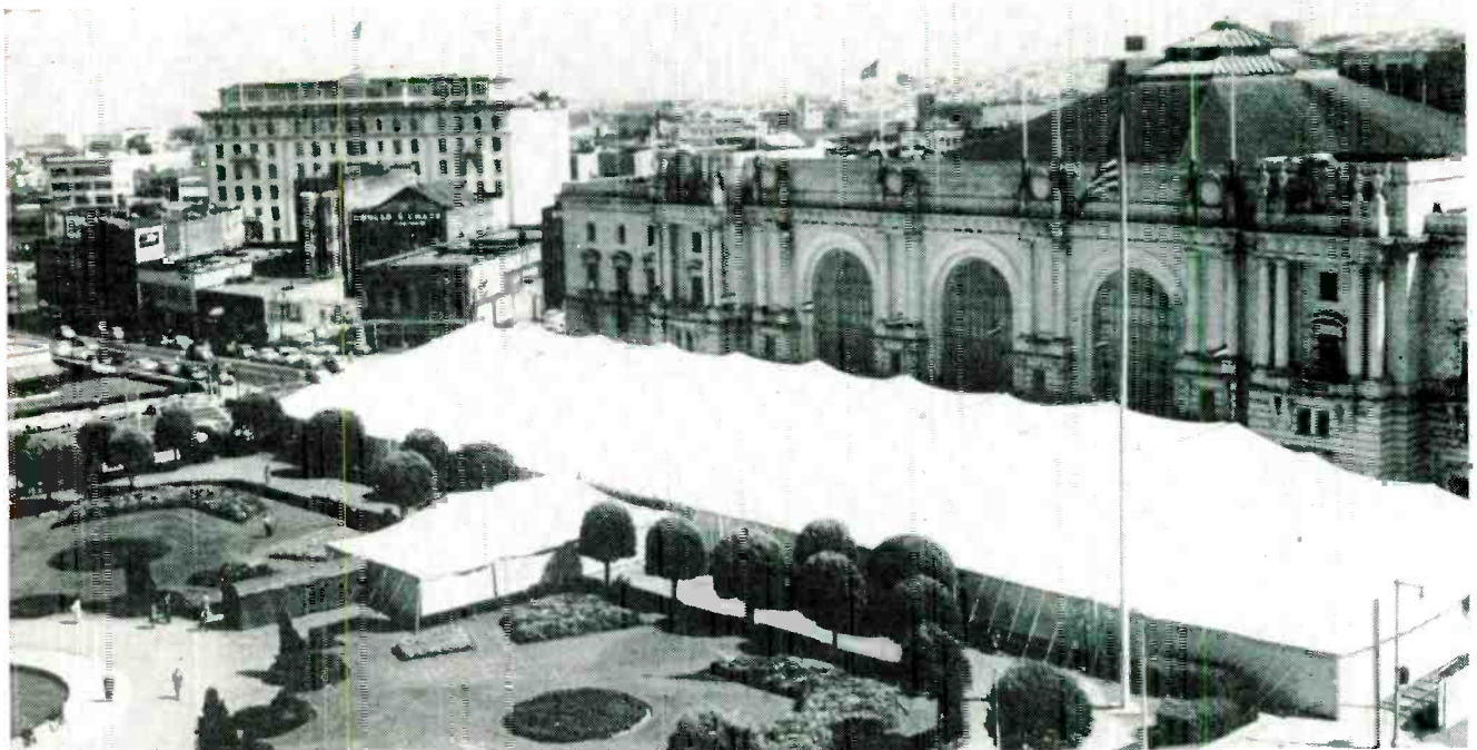
CIVIC AUDITORIUM in San Francisco will be the nation's electronic showplace when . . .
