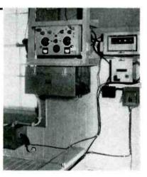
Interior installation at Barrett Rock control point. Antenna changeover switch is at upper right; radiotelephone receiver, with microwave transmitter mounted above, is at center. Antenna selector and transmitter controls are at left side of photograph
