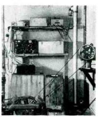
Interior installation at Holland Rock. On top shelf, from left to right, are: radiotelephone-transmitter control; time-sequence control; microwave receiver. Radiotelephone transmitter and batteries for receiver are below. Air compressor at lower left drives foghorn coding timer at right
