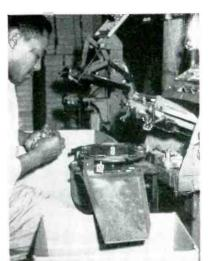
Selenium rectifier printing setup. Press operation and indexing are automatic, with speed being adjustable. Knockout bar has just pushed a stack out of turntable
