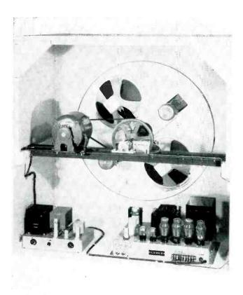
Loudspeakers are mounted on motor-driven baffle plate to produce pitch-fringing effect for realistic imitation of pipe organ
