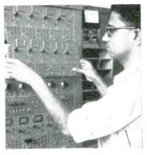
V. N. CHIPLUNKAR is shown installing an operational amplifier panel of a new computer recently built in the electrical communication engineering department of the Indian Institute of Science, Bangalore,
