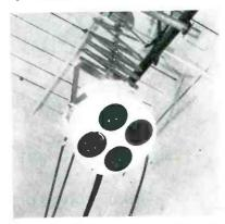
Multiplier phototube cluster picks up reflected light from objects hit by scanning beam. Two tubes have red filters; others pick up green and blue
