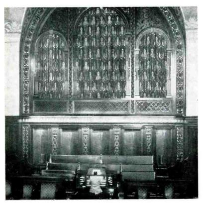
Installation of organ console in church. Loudspeakers are placed behind grill formerly housing organ pipes
