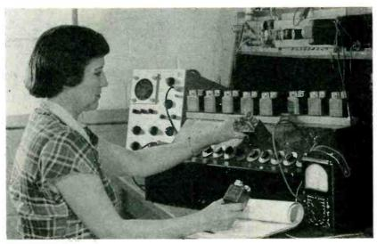
Production-line testing of plug-in type three-stage flip-flop counters
