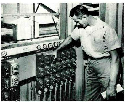
Operator on truck rack pushes button to select fuel. Lamps below buttons provide repeat-back and  $\bar{t}$ ailure-alarm information
