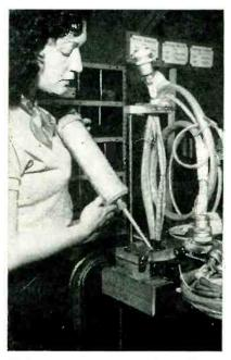
Filling steel radar assembly mold for large connector in Baltimore plant of The Glenn L. Martin Co.
