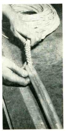
Guiding cable grip and conductors into tubing as operator at other end of tubing winds up cable on drum
