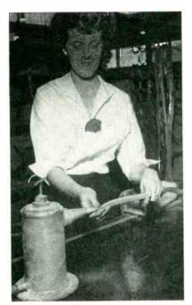
Setup for blowing talcum powder into plastic tubing to serve as lubricant. Threaded cap with T-shaped handle is removed from cylinder for refilling
