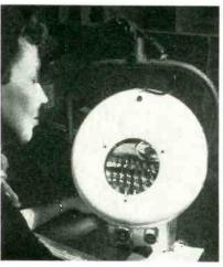
Magnification combined with intense illumination improves efficiency of inspecting screw terminals in missile black box
