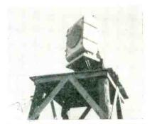
New packaged microwave telephone link mounted on platform for 50-mile circuit
