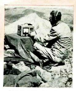
Taking antenna field strength readings atop 18,783 ft. Mt. McNamee.
