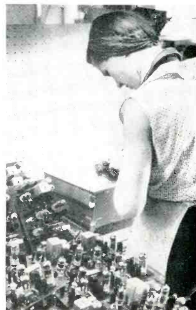
Dip-soldering assembled boards manually. Solder pot has positioning pegs to insure correct depth of immersion
