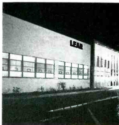
Lear's new Santa Monica plant
