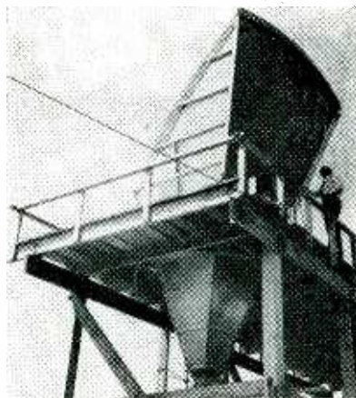
Horn-reflector antennas resembling giant sugar scoops have been designed by Bell Labs for use on radio relay routes. The new antennas may eventually handle up to 20,000 telephone circuits or 30 tv programs at one time
