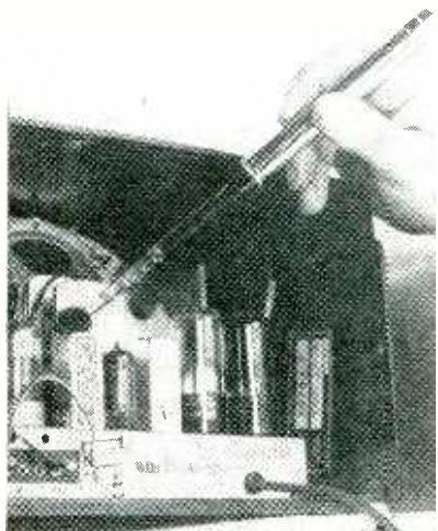
Inspecting top of transformer without removing chassis from cabinet. Mirror provides 1½-times magnification
